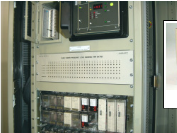
Tripping Matrix Power Control
