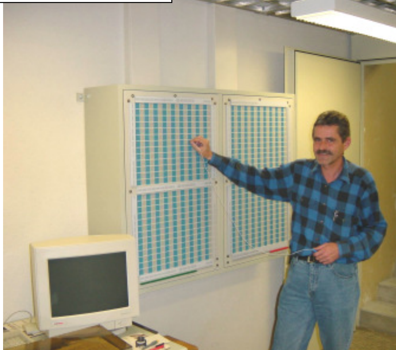
GKVA 200x210 314 LA K, Telecom Matrix 2-pole for routing of data and telecom signals
