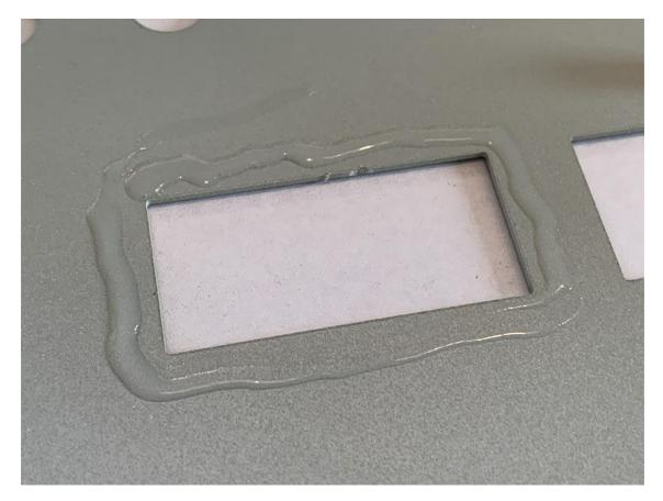
Before the glue dries, simply place the red label as centrally as possible over the opening and press it on gently. Make sure that the middle of the shield is not smeared with glue! The best thing to do is to simply lay it on the fresh glue and let it dry.
